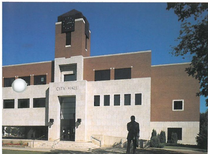
Project: CITY HALL — Prince Albert, Saskatchewan Architects: Wiens Architects na, Saskatchewan Stone: Buff, Sawn and Rubbed finish cut dimension stone
