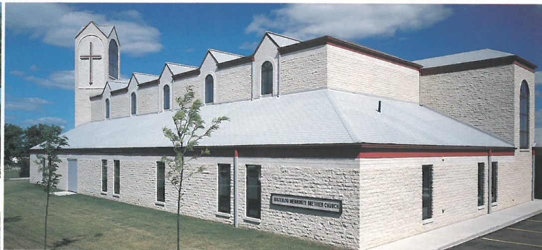
(ABOVE) Project: WATERLOO MENNONITE BROTHERS CHURCH — Waterloo, Ontario Architects: Turhan Okeren Architect Ltd. — Saskatoon, Saskatchewan / Maurice van Nes-Waterloo, Ontario Stone: Grey, Split-Face and Sawn-Face random ashlar
