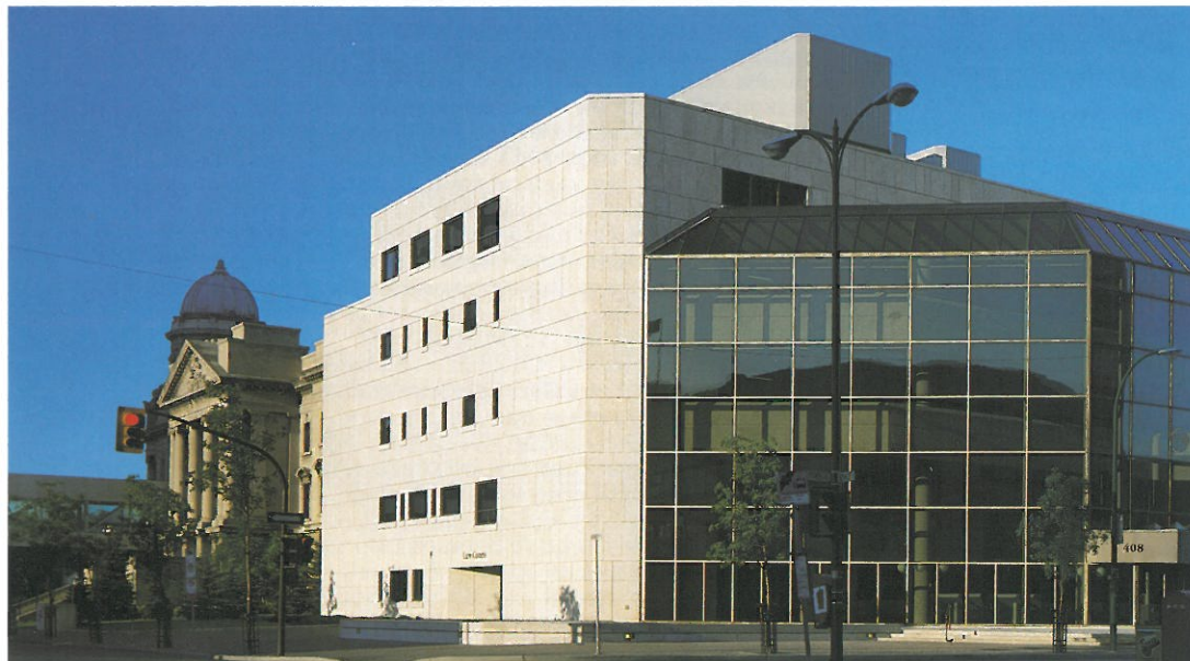
(ABOVE) Project: LAW COURTS BUILDING — Winnipeg, Manitoba Architects: Number Ten Architectural Group — Winnipeg Stone: Buff, Sawn finish cut dimension stone
