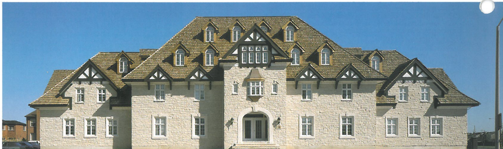
(ABOVE) Project: JOHN BODDY DEVELOPMENTS LTD. HEAD OFFICE BUILDING — Scarborough, Ontario Architects: Deacon Arnett Murray & Rankin — Agincourt, Ontario Stone: Buff, Three-Course Split-Face random ashlar machine pitched, and Buff, Rubbed finish cut dimension stone trim
