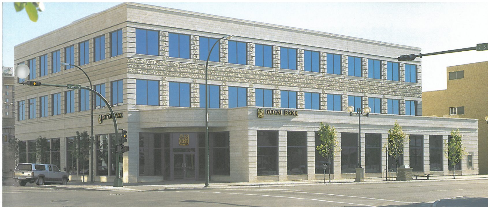
(ABOVE) Project: ROYAL BANK OF CANADA BUILDING — Lethbridge, Alberta Architects: The Cohos Evamy Partnership — Calgary, Alberta Stone: Buff, Split-Face machine pitched and Sawn-Face Random Ashlar, and cut stone
