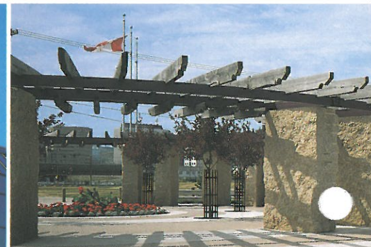
(ABOVE) Project: ORIENTATION NODE THE FORKS NATIONAL Arch. Ptnrshp (Ldsepg) Hilderman Witty Crosby Hanna Assoc. Stone: Buff, Rubbed finish cut dimension stone
