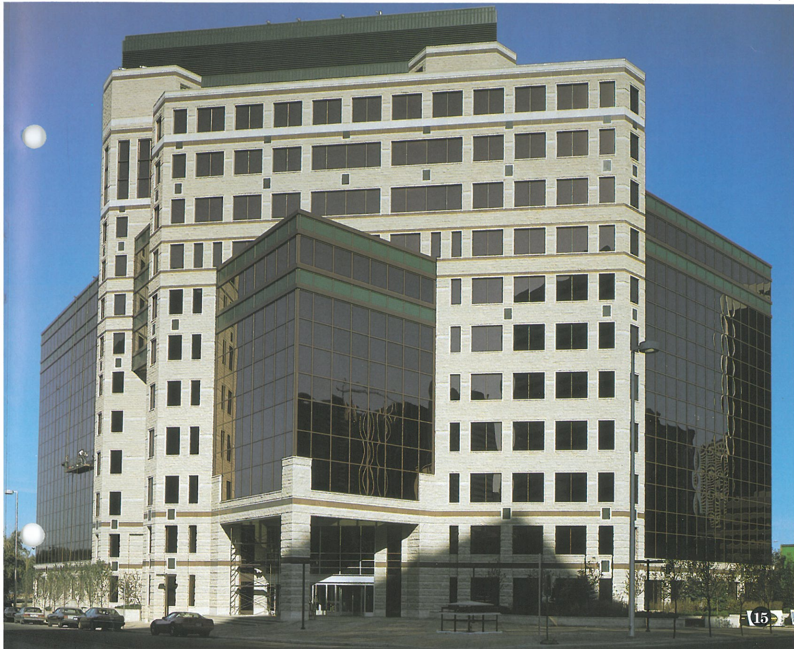
(BELOW) Project: SHELL CANADA LTD. OFFICE BUILDING — Calgary, Alberta Architects: The Cohos Evamy Partnership — Calgary, Alberta Stone: Grey, Split-Face and Sawn-Face Random Ashlar, and cut stone
