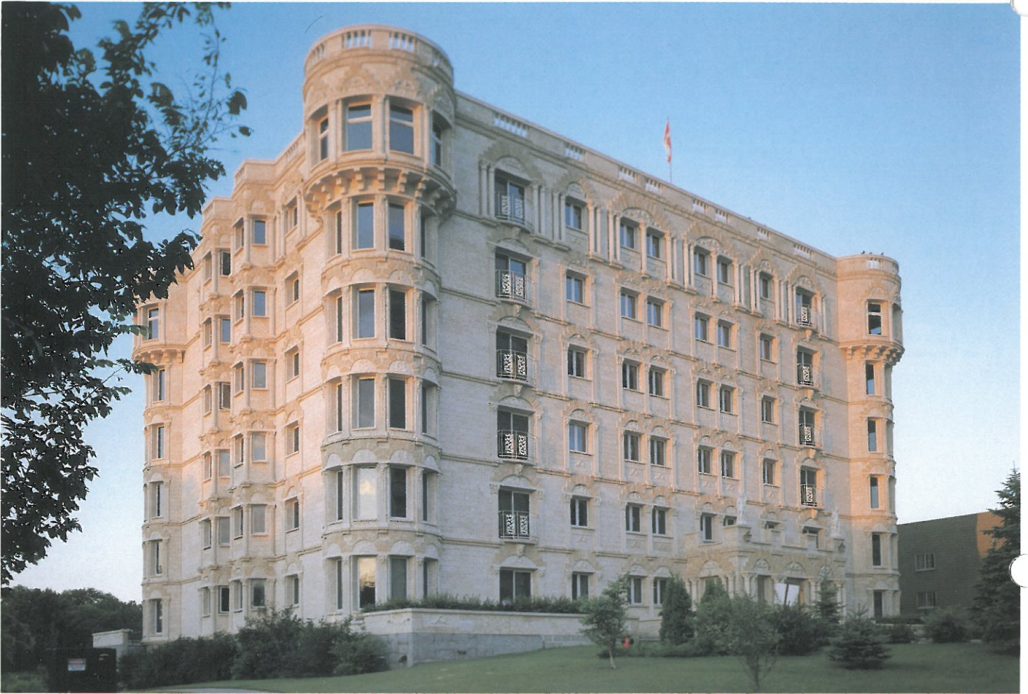
Project: CASTLE ON THE SEINE — CONDOMINIUM APARTMENT BUILDING — Winnipeg, Manitoba Architects: MMP Architects — Winnipeg, Manitoba Stone: Golden Buff, Sawn-Face and Split-Face random ashlar. Sawn sills, soffits, copings. Rustic-Face arches.
