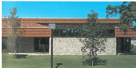
Project: LIBRARY — North Battleford, Saskatchewan Heetham & Rattan Architects — North Battleford, Saskatchewan Red Color, Split-Bed Rustic LedgeStone "Dry-Pack" random ashlar
