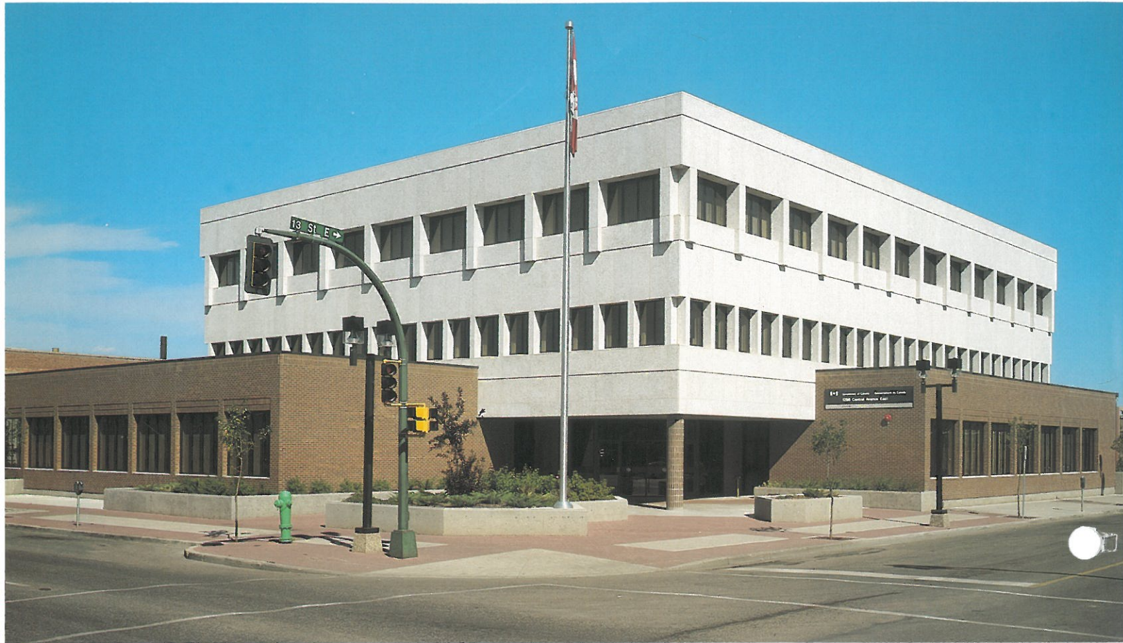
Project: GOVERNMENT OF CANADA OFFICE BUILDING — Prince Albert, Saskatchewan Architects: Scott Bowers Architect & Engineer — Saskatoon, Saskatchewan Stone: Grey, Rubbed finish, cut dimension stone.
