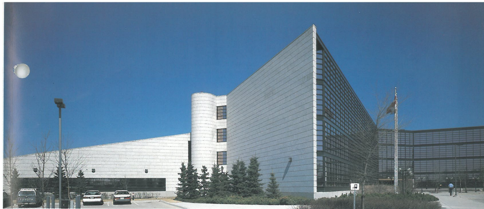
(ABOVE) Project: AIR COMMAND HEADQUARTERS BUILDING — Winnipeg, Manitoba Architects: Aircom Consultants — Winnipeg, Manitoba Stone: Grey, Sawn finish cut dimension stone panels
