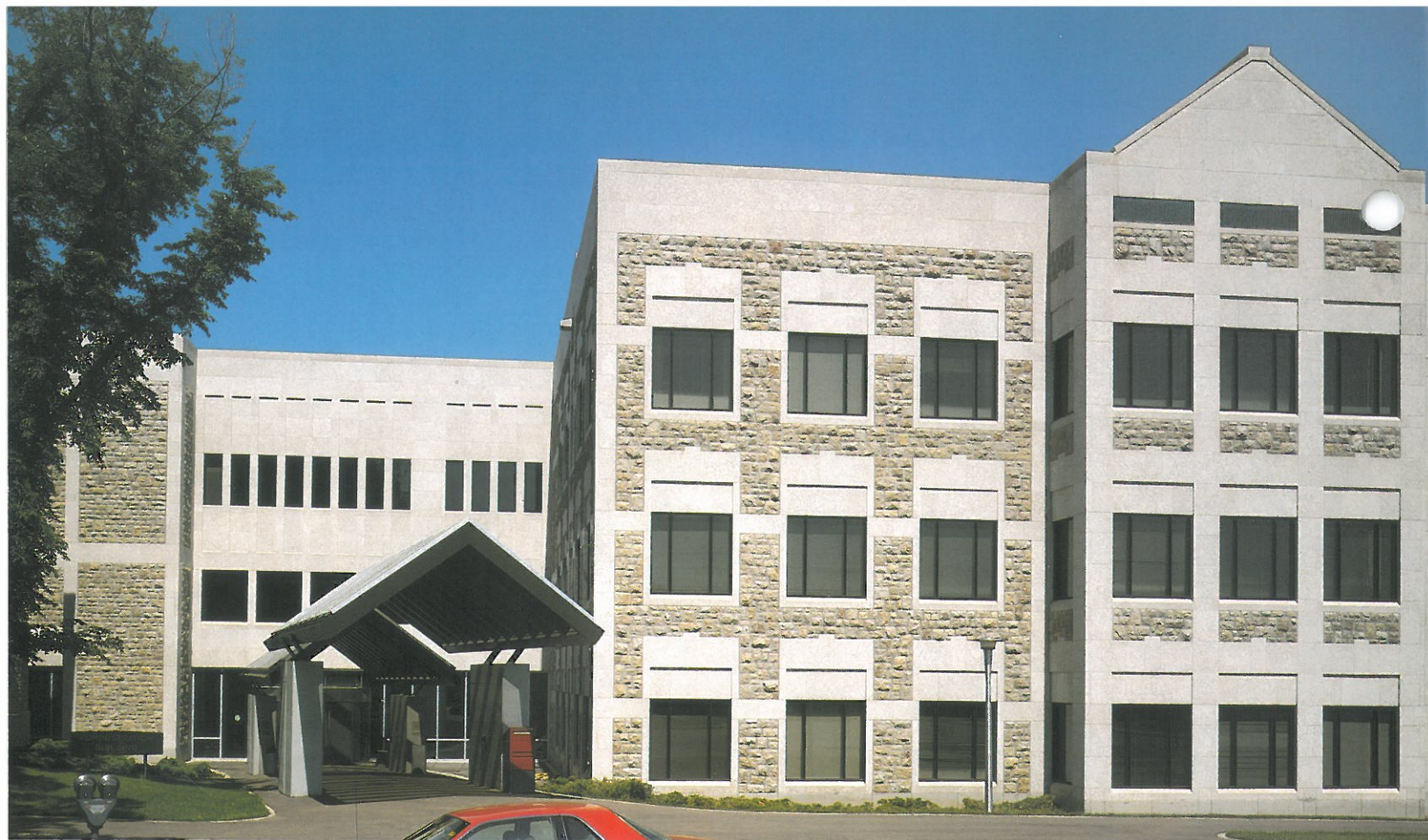
(ABOVE) Project: ADMINISTRATION BUILDING, UNIVERSITY OF SASKATCHEWAN — Saskatoon, Saskatchewan Architects: Wiens Architects Ltd. — Regina, Saskatchewan Stone: Buff, Sawn finish, cut dimension stone
